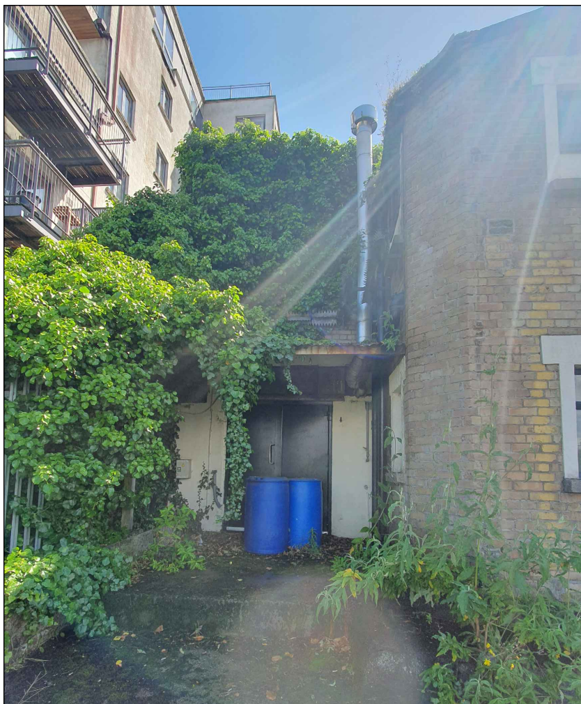
EXISTING NORTH ELEVATION Disused Office Building
