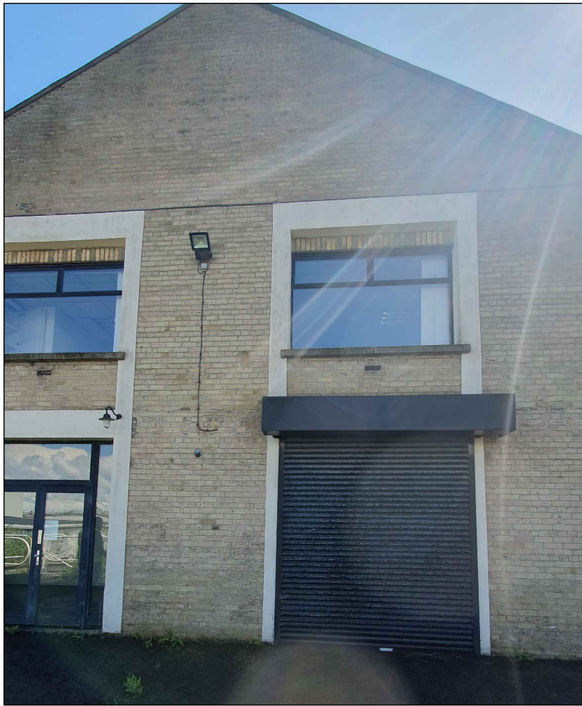
EXISTING NORTH ELEVATION Disused Office Building
