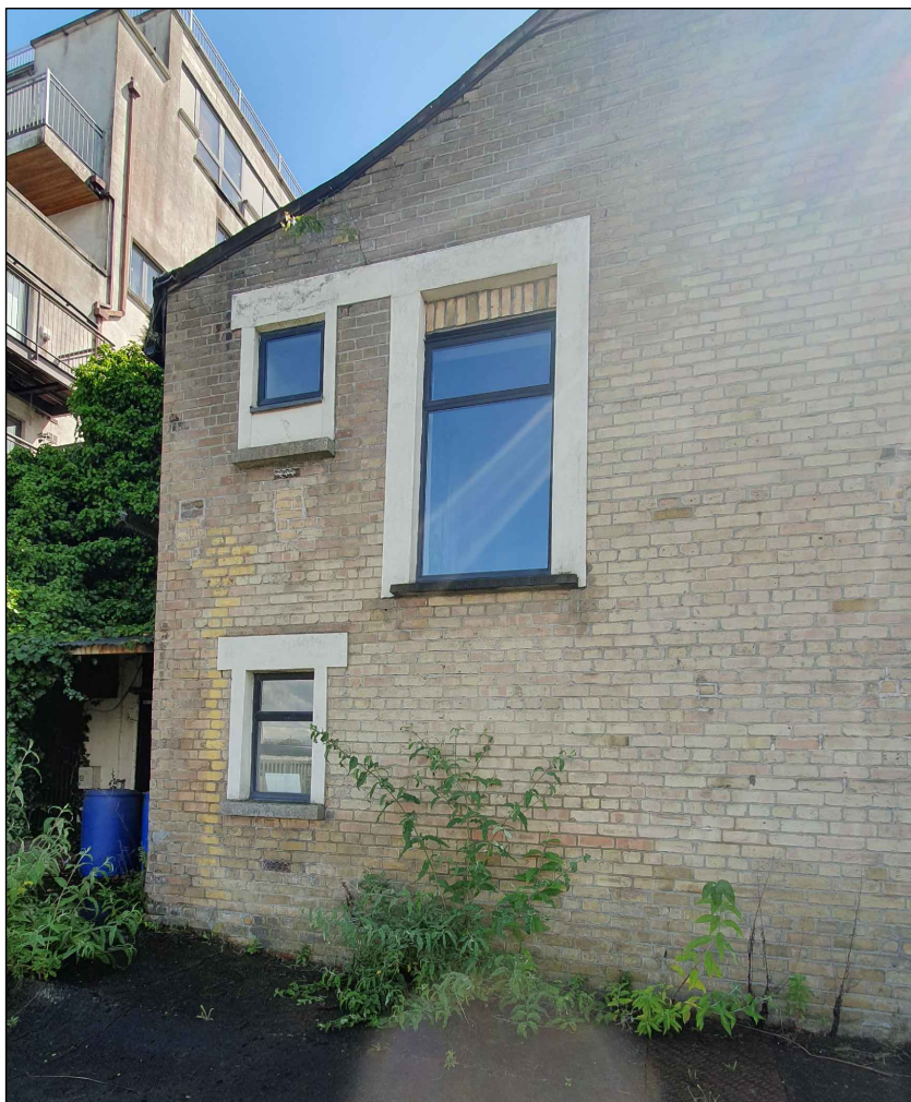
EXISTING NORTH ELEVATION Disused Office Building
