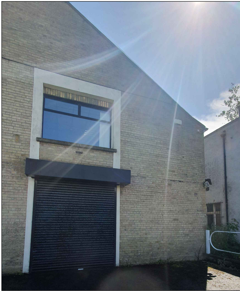
EXISTING NORTH ELEVATION Disused Office Building
