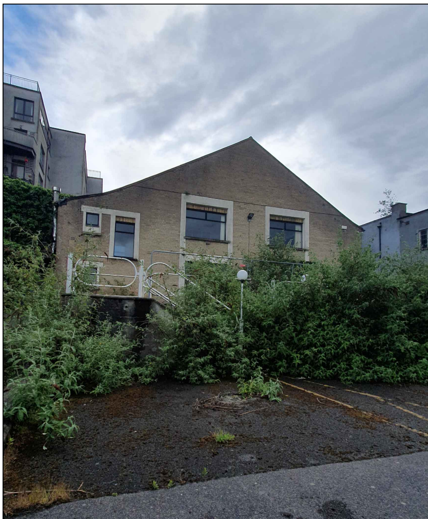
EXISTING NORTH ELEVATION Disused Office Building
